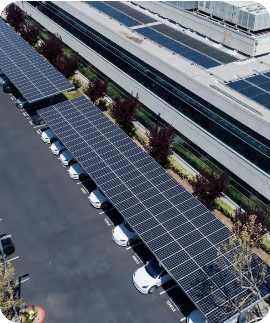
MPS San Jose offices, USA
