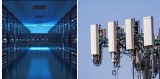
Datacenter & 5G Backup
